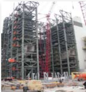
Boiler structural steel is erected at Trimble County Unit 2.
