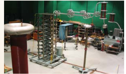
The Ohio State University High-Voltage Laboratory
